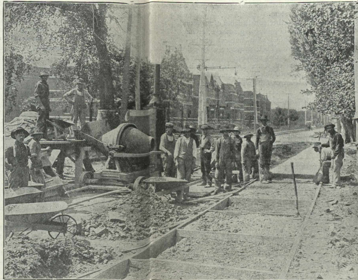
Smith Concrete Mixer on Sidewalk Work
