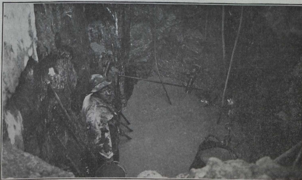
Sinking Shaft on Gold Quartz Vein at Burnside Mine, Kirkland Lake, Ont.
