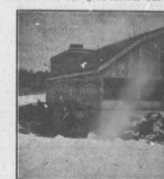
A House Designed to House a Farm Flock Larger Than the Average. This 20 x 30-foot house will accommodate housing this number of birds in one flock and in this style of house is now being investigated at the Ontario Agricultural College poultry department, where this photo was taken by an editor of Farm and Dairy approaching the house is Mr. Robert Essex, one of the well known poultry men of the United States.
