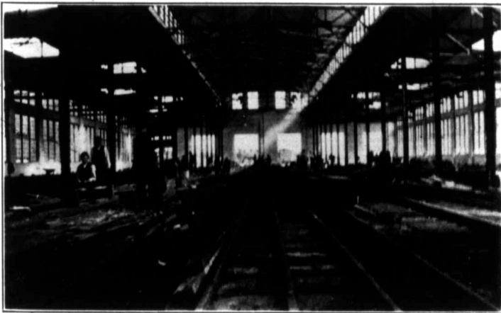
Interior of Freight Car Shop.
