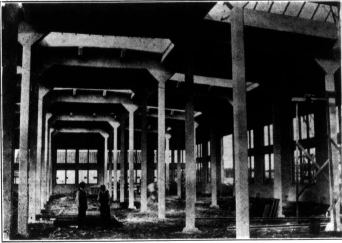
Interior of Passenger Car Shop.
