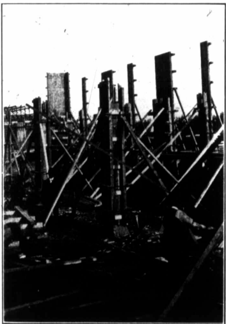
Columns for Mezzanine Floor, Passenger Car Shop.
