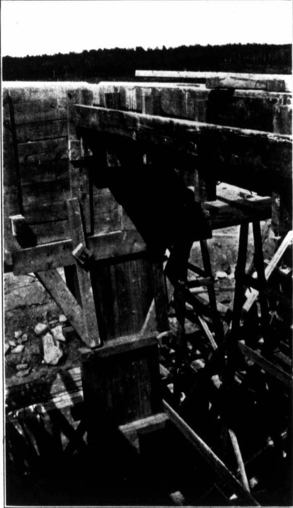
Forms for Beams, etc.
