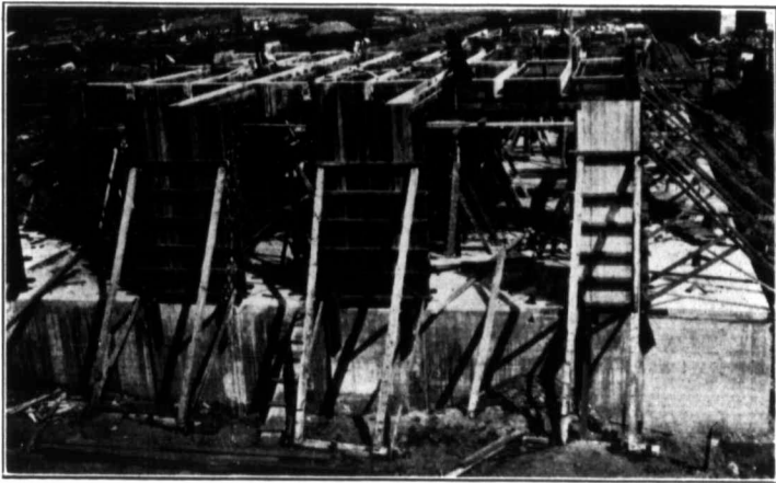
Forms for Second Story, Stores and Office Building.
