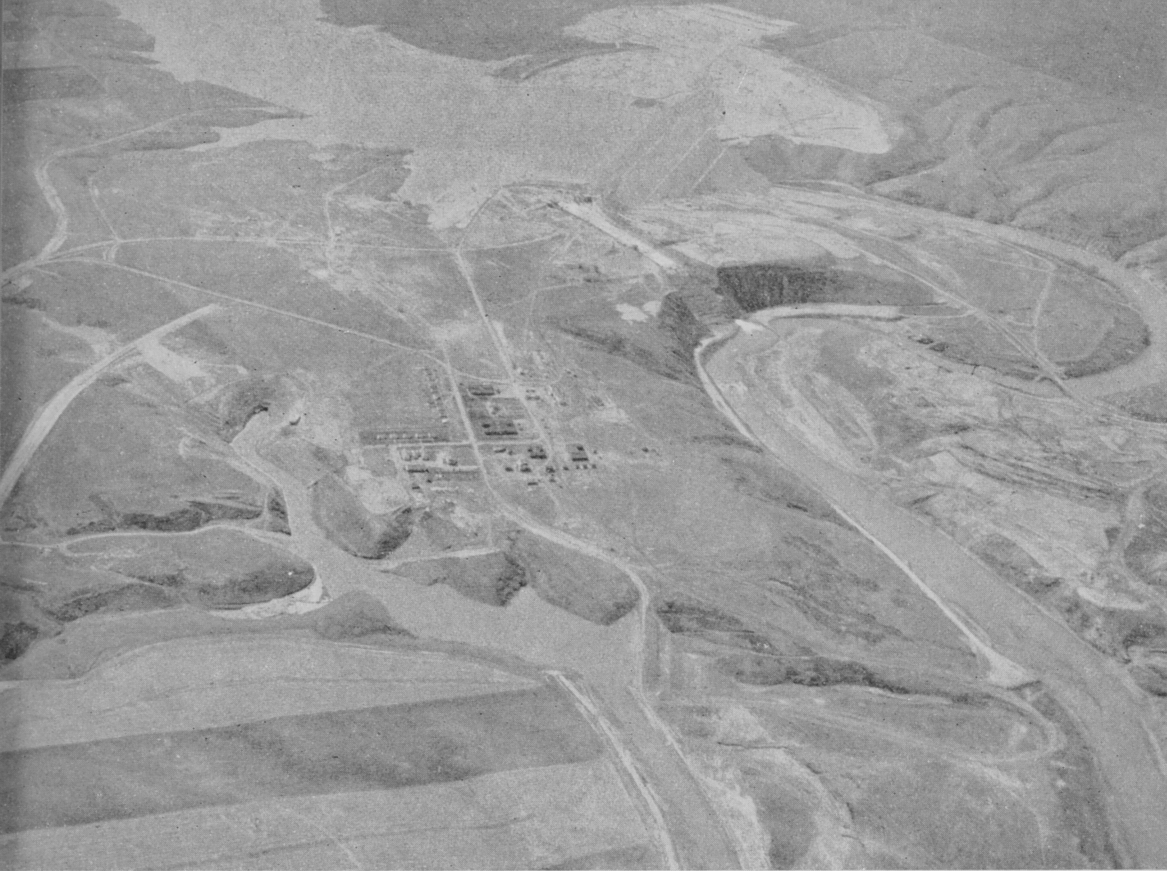
An aerial photograph of the St. Mary Dam.
