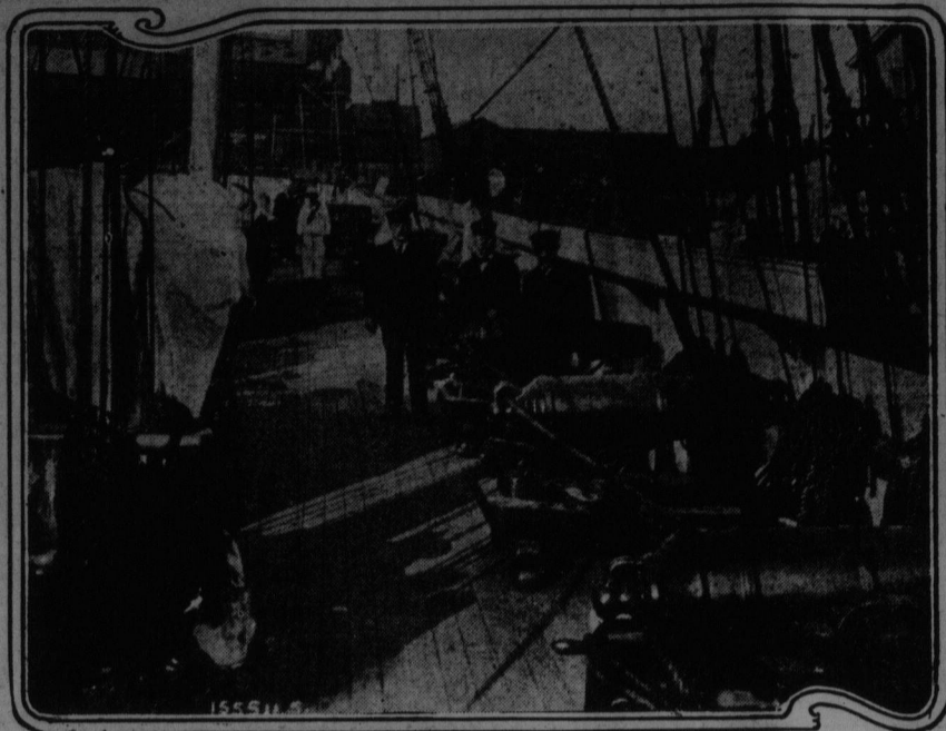
The above photograph shows part of the gun deck of the rebuilt Niagara, Commodore Perry's flagship. The vessel was launched at Erie, Pa. The old war brig was used to commemorate the centennial of Perry's sweeping victory at Put-In-Bay.
