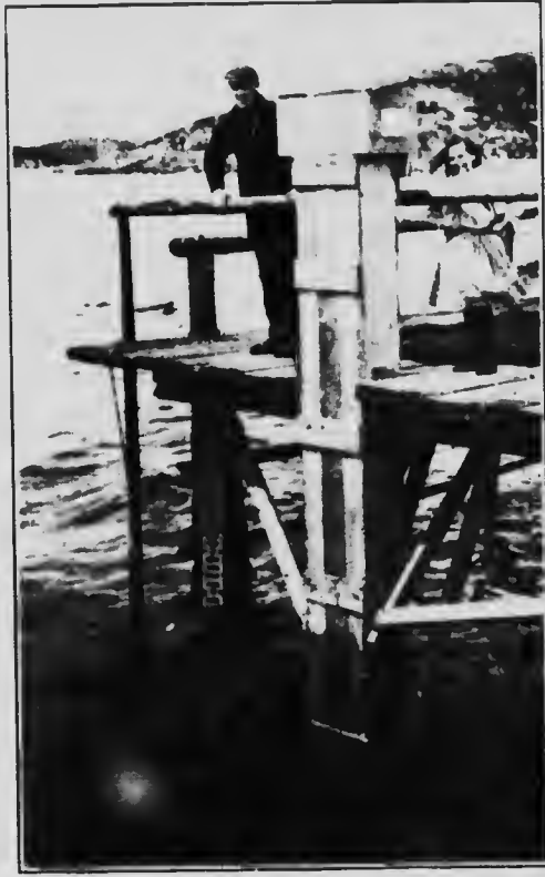
TEMPORARY TIDAL STATION showing a scale and tide column with shelter box on top which contains the Recording Instrument.
