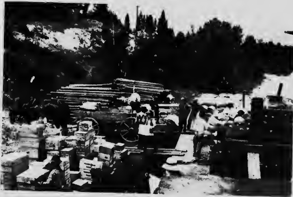
Unloading Camp Supplies on Company's Property
