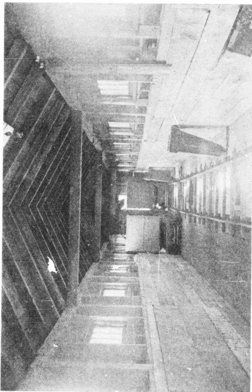
Elevated Floor for Roasted Concentrates.—Brookfield Chlorination Works, Nova Scotia.
