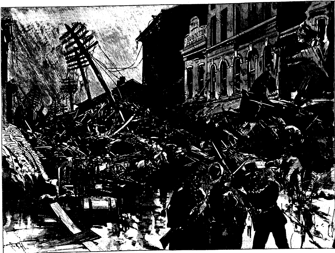
THE JOHNSTOWN FLOOD.—MAIN STREET, JOHNSTOWN, AFTER THE FLOOD.
