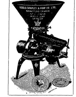
is supplied with two sets of Grinding Burrs, one for coarse grain and general purposes, and the other for hard grain and fine work.
