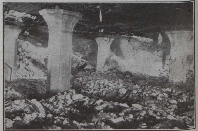
Fig. 13—View in Basement Where Premiums Were Stored.
