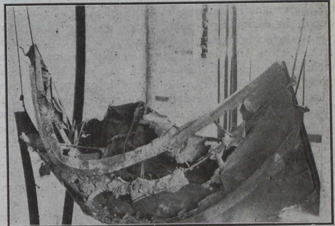
Fig. 15—Tin-Clad Wooden Fire Doors Were Practically Useless.
