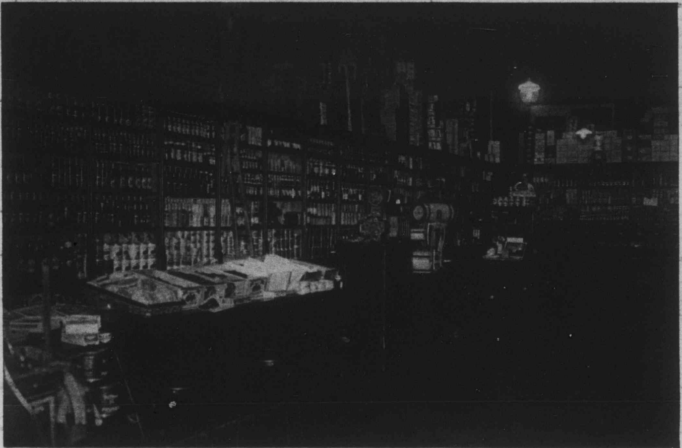
The attractive store interior of A. L. Pinard, Rideau Street, Ottawa.
