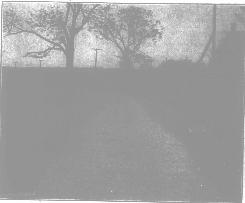
Crushed Stone Left Unrolled.
