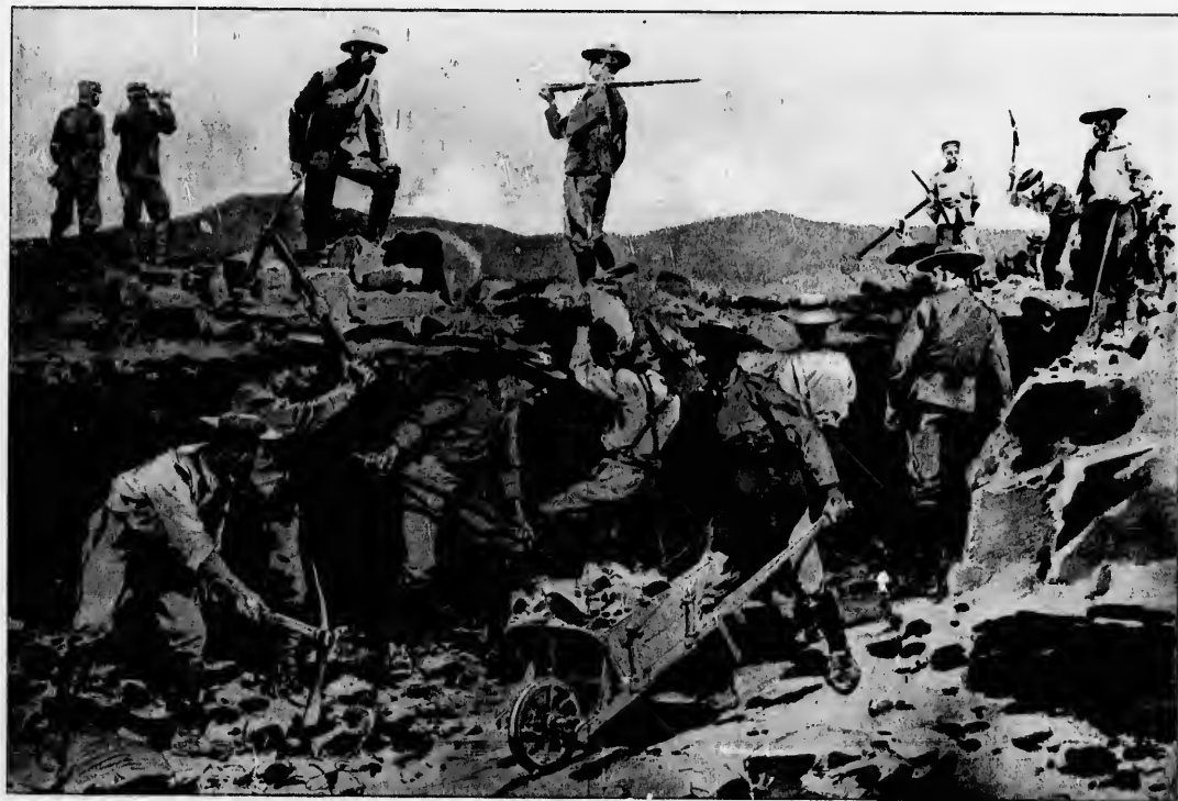
THE BLUE-JACKETS IN THE TRENCHES. —When the sailors in the British navy were landed in South Africa to help raise the siege of Ladysmith they found unusual employment from the first. The Boers had entrenched themselves among the mountains and "kopjes" surrounding and overlooking Ladysmith, whence they could throw a destructive fire at any force coming within range. This made it necessary for the blue-jackets to dig trenches and throw up breast-works from the start. The artist has happily illustrated the method of performing the work, and has presented a clear idea of the difficulty and hardship connected with the labor, owing to the rocky condition of the soil in many places. The rocks and clay, so common to the soil in South Africa, made good breast-works that stopped many a Boer bullet.
