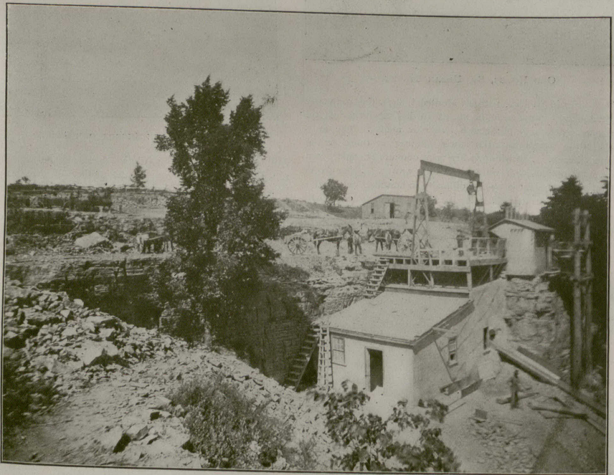
VIEW OF CRUSHER AT DOOLITTLE & WILCOX QUARRY, DUNDAS ONT.
