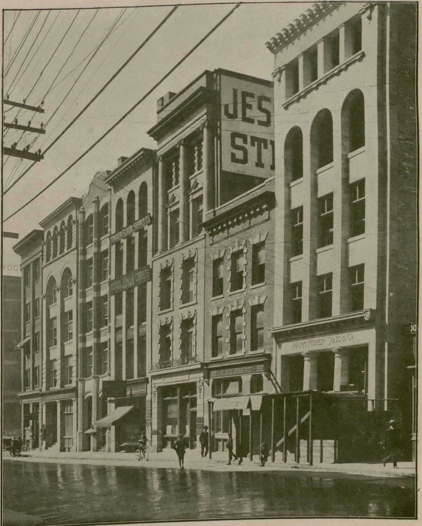
REBUILDING THE BURNED DISTRICT IN TORONTO. WAREHOUSES ON BAY STREET.
