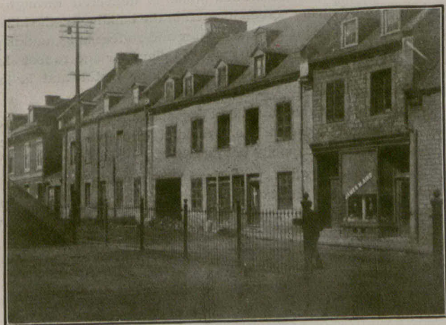
OLD HOUSE, ST. URBAN STREET.
