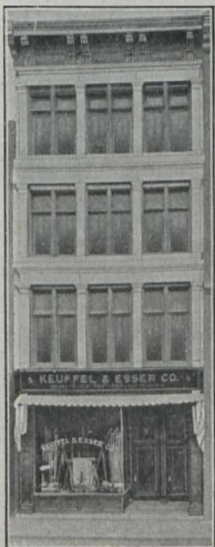
K & E Building, Montreal
