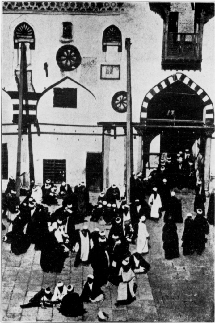
INTERIOR OF MAIN COURT, EL AZHAR UNIVERSITY, CAIRO. Showing the dilapidated condition of the building.
