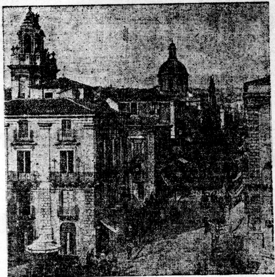
Main Street in Reggio, destroyed by the earthquake. The cathedral, of which the dome is shown, was completely wrecked, with the rest of the city.
