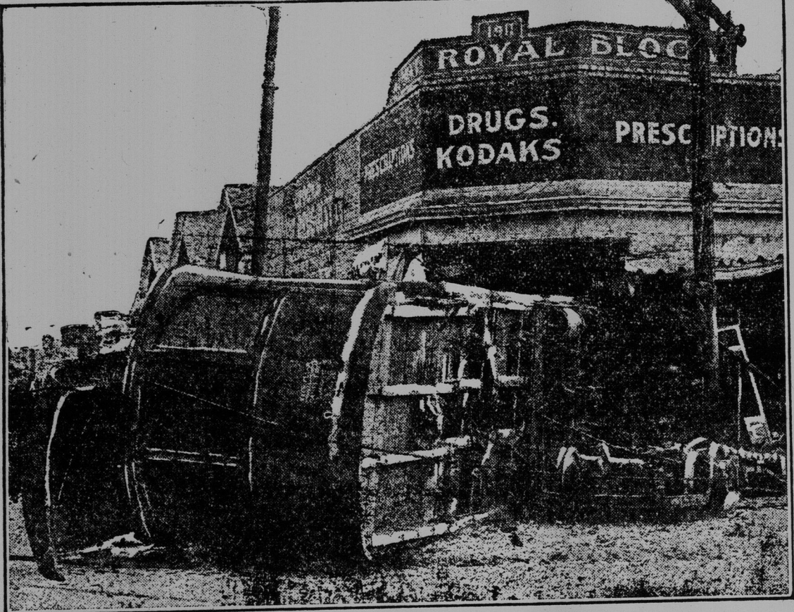
Caused $22,408 damage at Calgary where three killed and dozen injured.
