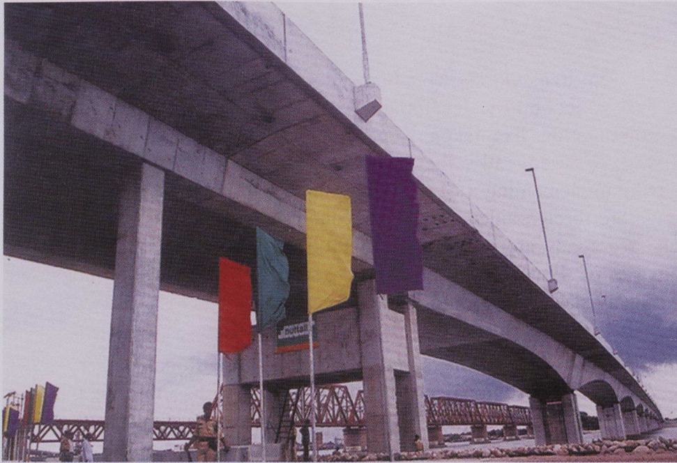
Bridge over the river Meghna on Dhaka-Sylhet Highway
