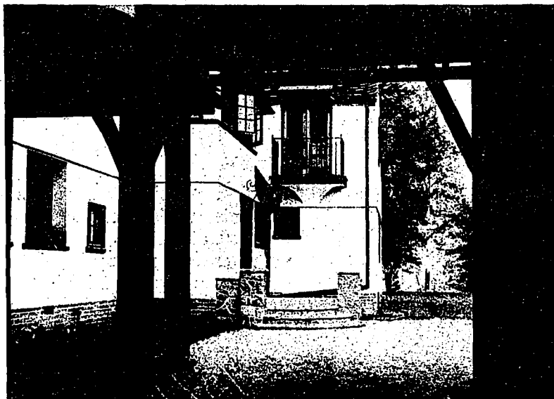
DRIVEWAY APPROACH TO ENTRANCE.
