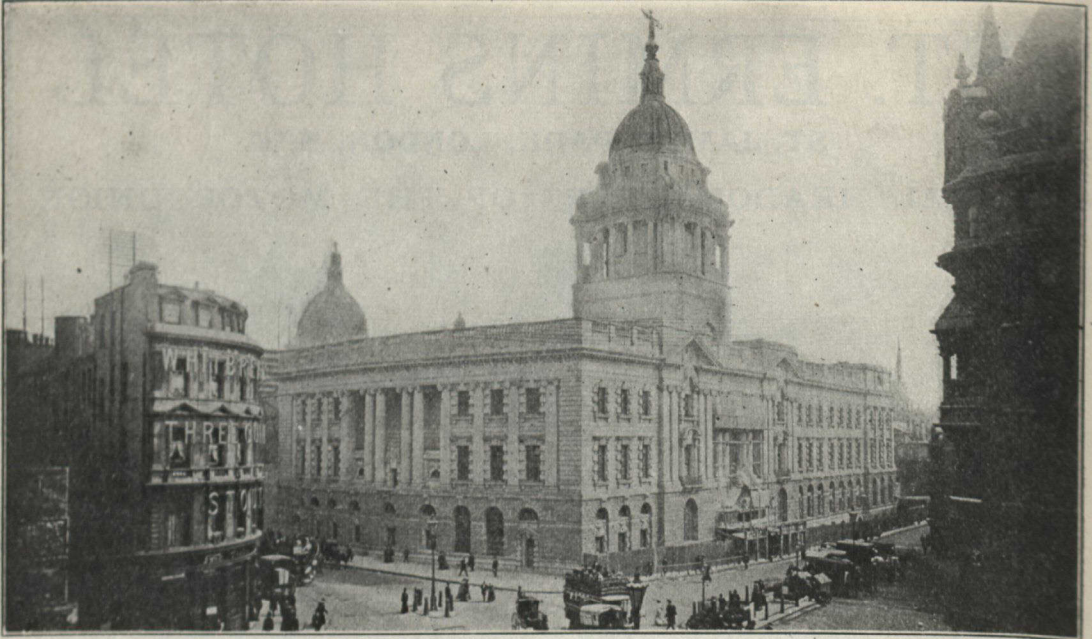
The new Bailey is worthy of the greatness of modern London and takes rank with the great palaces of justice for which Europe is celebrated. Frontage, 287 ft. (Old Bailey) and 142 ft. (Newgate St.); average height from pavement to top of balustrade, 75 ft.; height of dome to the ball, 195 ft.; bronze figure of Justice, 12 ft. high; civic sword held by statue, 6 ft. long. Figures over entrance representing "The Recording Angel," "Truth" and "Fortitude," sculptured by Mr. F. W. Pomeroy, A.R.A.
