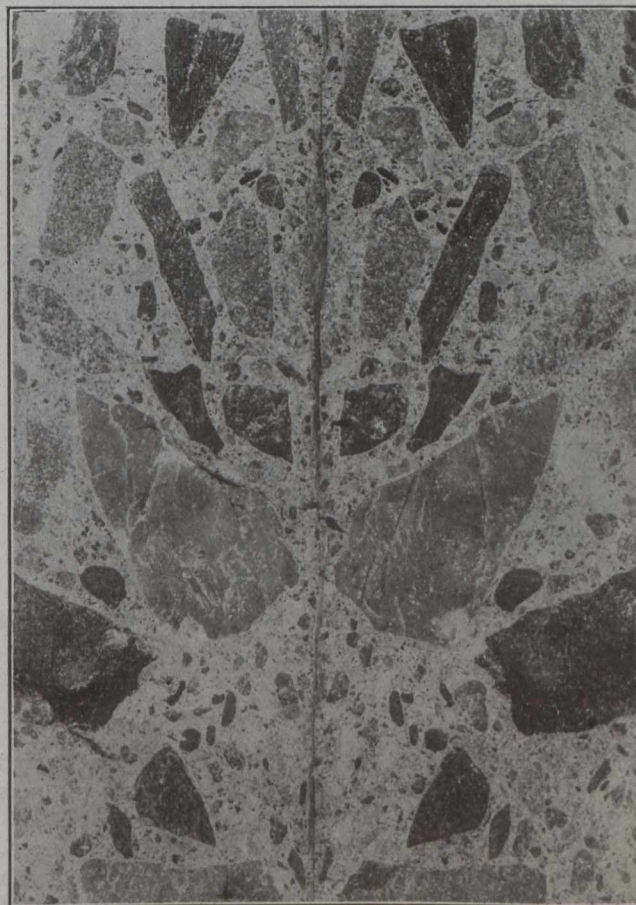
Fig. No. 26.—Fractured Concrete; 1:2:4 Mix; First Consistency ( \times 1\frac{1}{2} )
