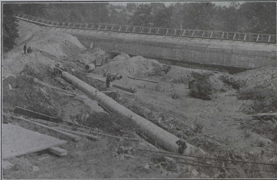
Woodville Avenue Sewer Complete and 3-foot Concrete Pipe
