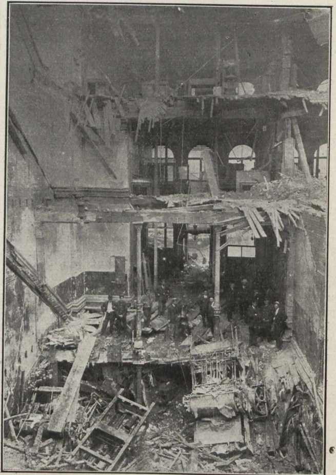
Showing the Clean Cut Through Floor
