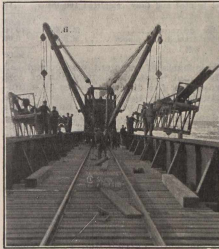
Fig. 7—Method of Raising and Moving Rivetting Galleries.
