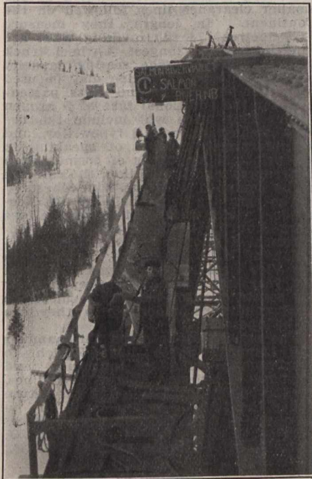
Fig. 8—Rivetting Gallery in Position at Top Tower.
