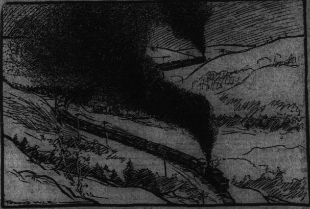
ed by making a double curve; the road crosses the creek at a low point where very little filling is required. A wooden trestle spans the gap. These features entail the use of a "pusher" engine, a w rate of speed and a vast consumption
