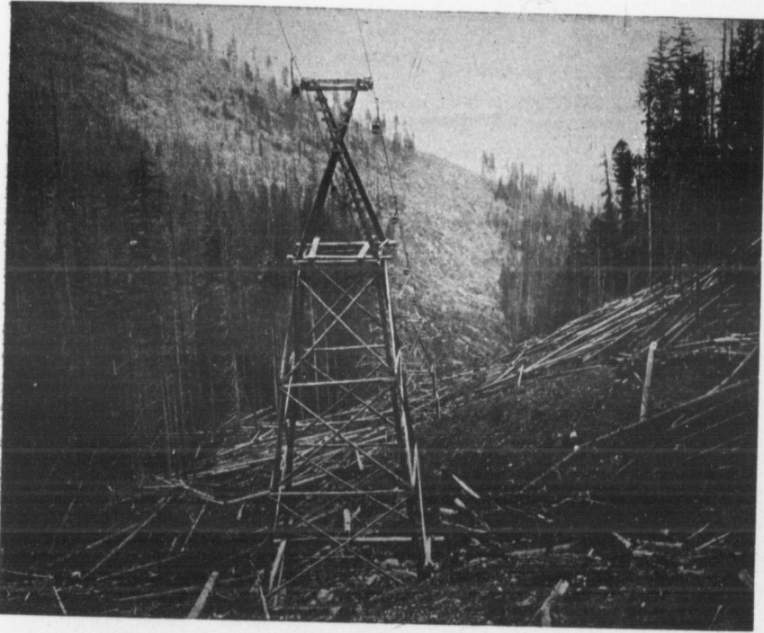
RAISED A X TOWER ON SINGLE ROPE CABLEWAY.
