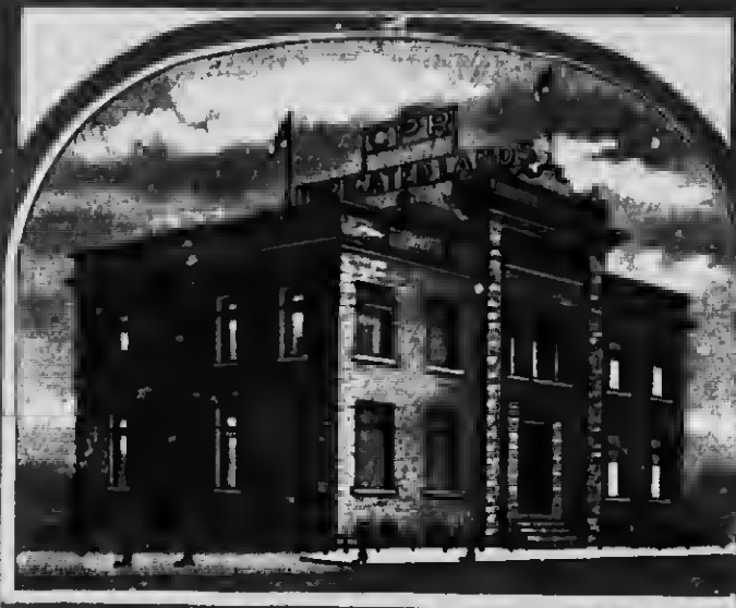
OFFICE BUILDING OF THE COMPANY CALGARY, ALBERTA
