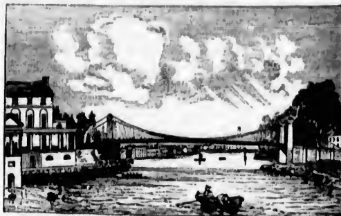
Wire Bridge over the Schuylkill river, with part of Fairmount.
