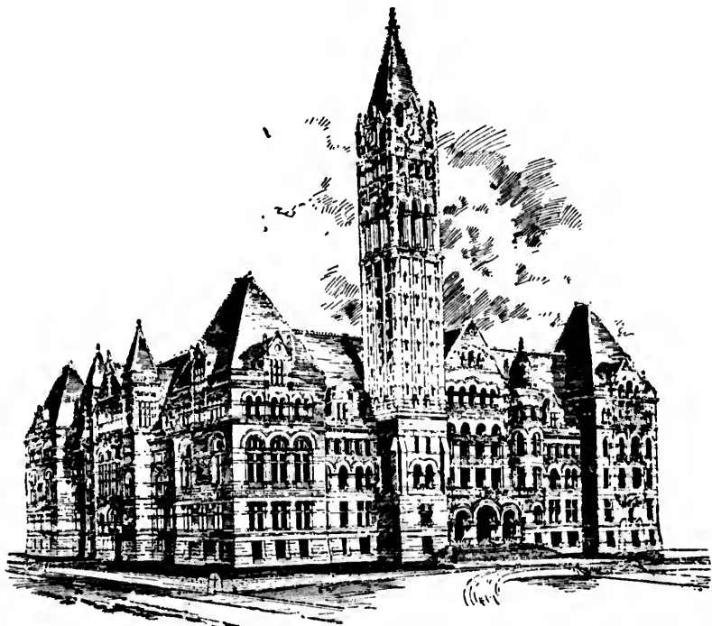
CITY AND COUNTY BUILDINGS (UNDER CONSTRUCTION), TORONTO.
