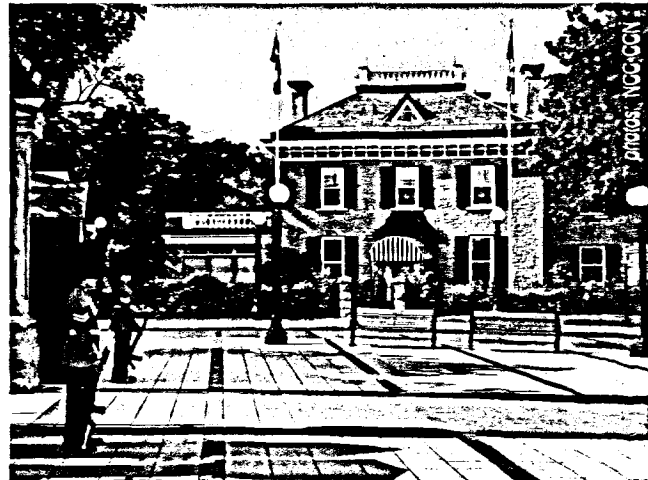
With all its exuberance stripped away, 7 Rideau Gate today presents a dignified, Georgian face.
