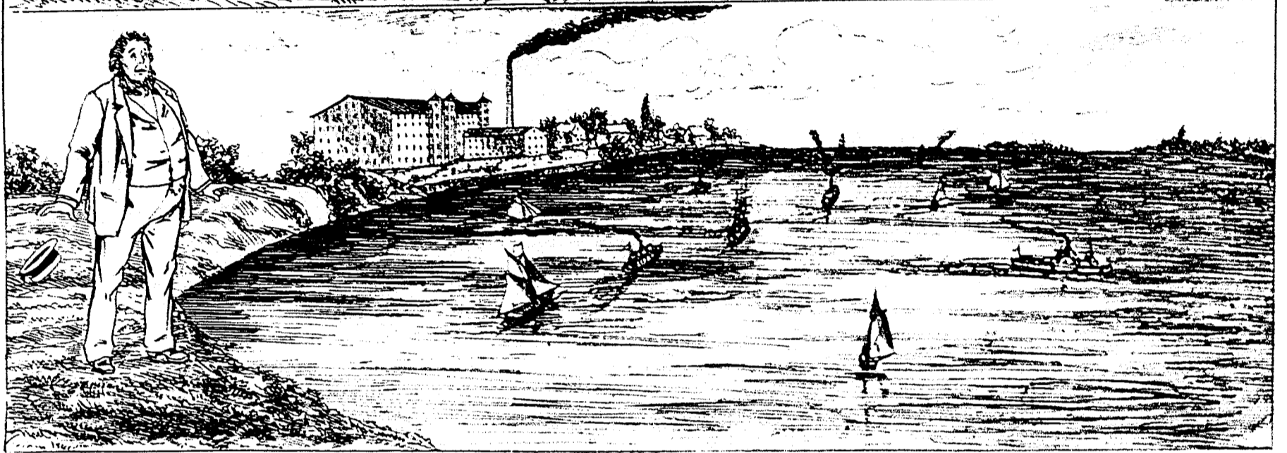
THE TUNNEL ACROSS THE ST. LAWRENCE AT MONTREAL.—A DREAM AND THE REALITY.
