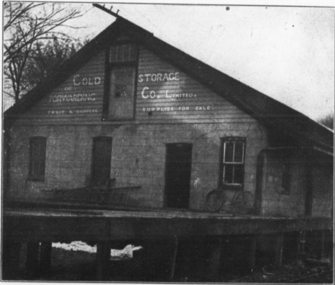
St. Catharines Cold Storage Company.
