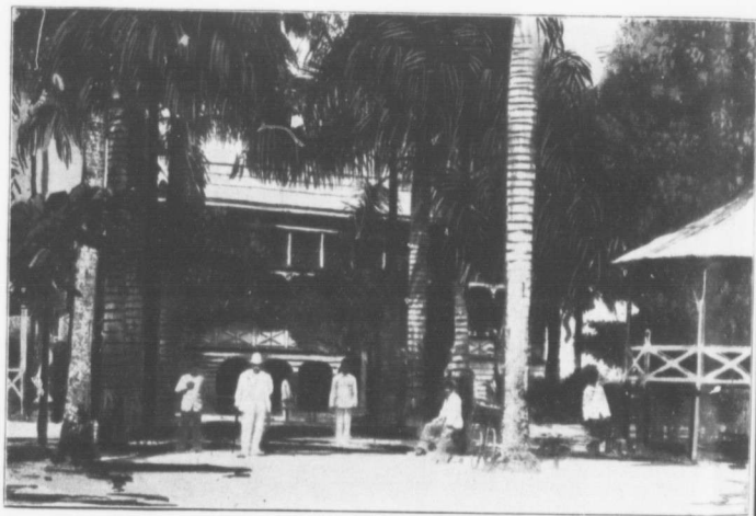
DUTCH GUIANA.—Club House "Het Park."
