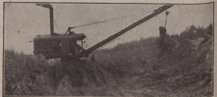
Drag-line Excavating Aqueduct Trench
