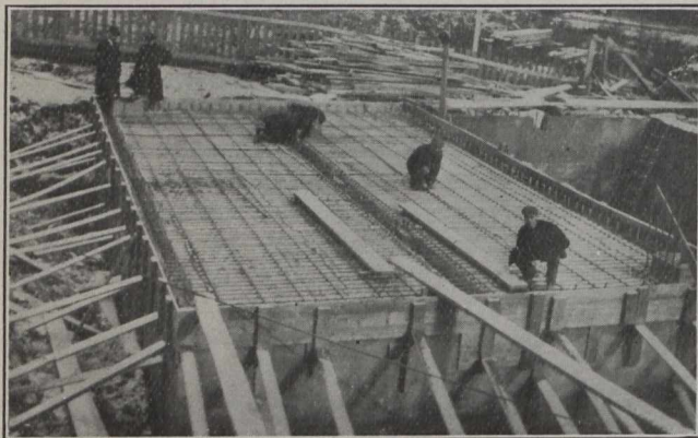
View of Tanks, Showing Reinforcement.
