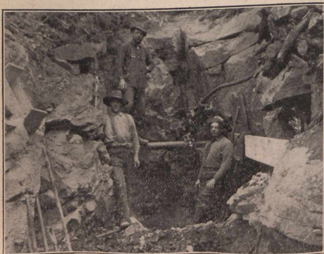
ROCK DRILL IN CUTTING, WHITE MINE.
