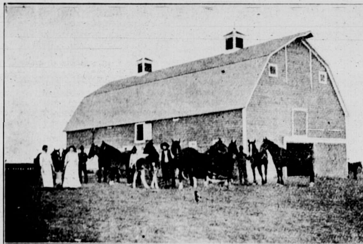
A Substantial Barn on the farm of James Caulder, Pasqua, Sask.
