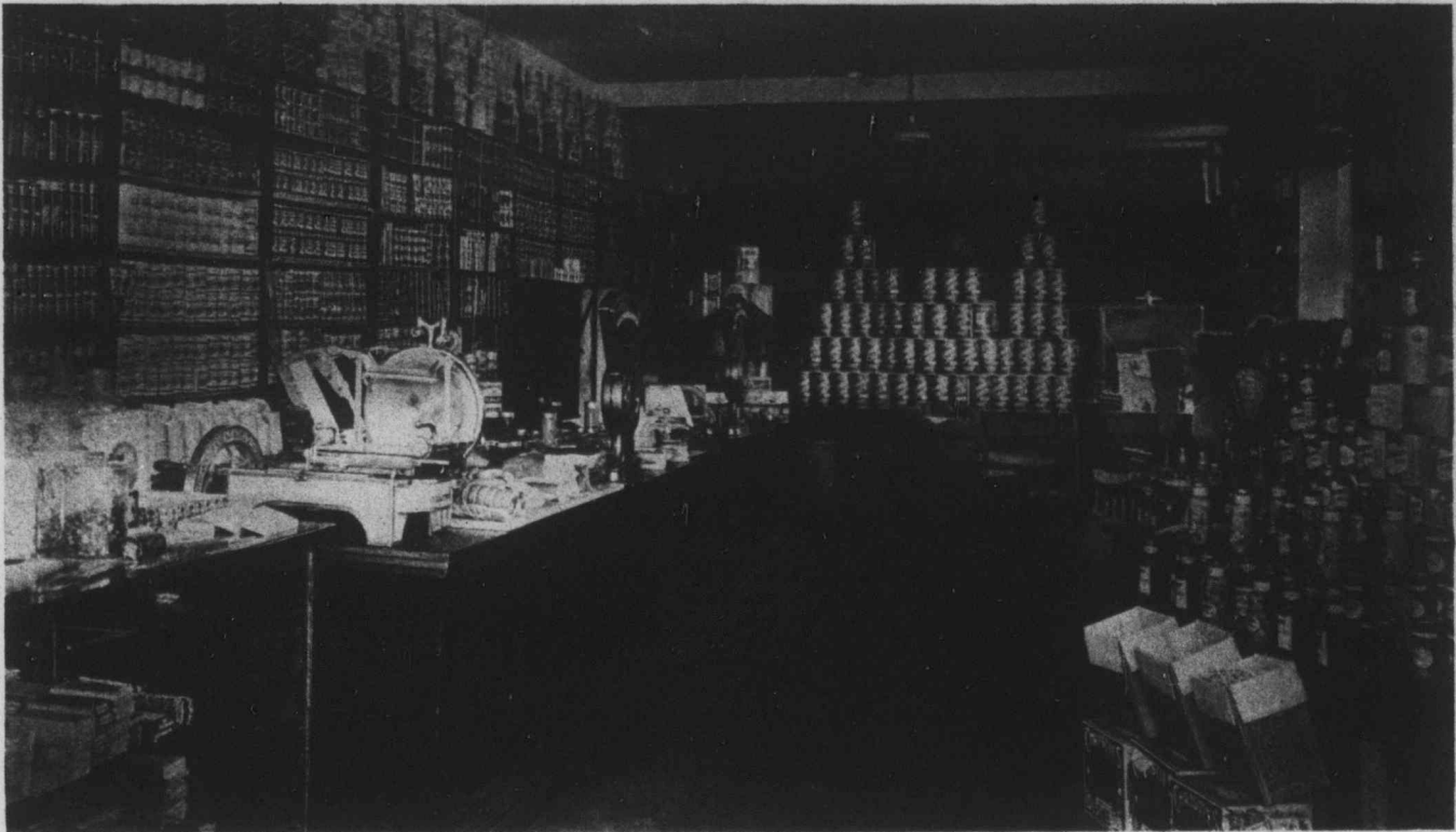
An attractive grocery interior. The Ferguson Store, Queen Street East, Toronto.
