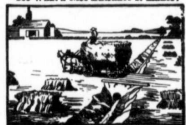
Best Culvert for the Fields!
