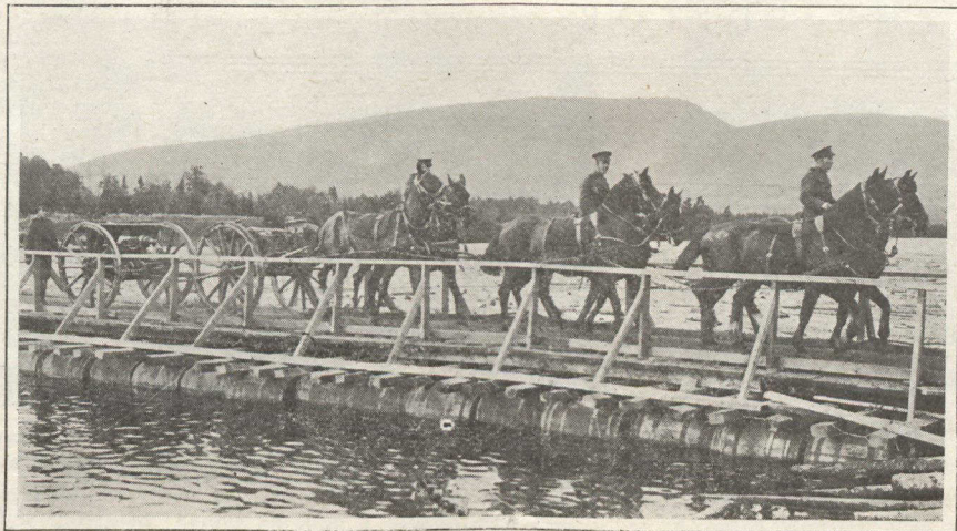
A pontoon bridge of coal-oil barrels and planks over the Jacques Cartier River and a gun of the 13th Battery, St. Catharines, on the way over it.
