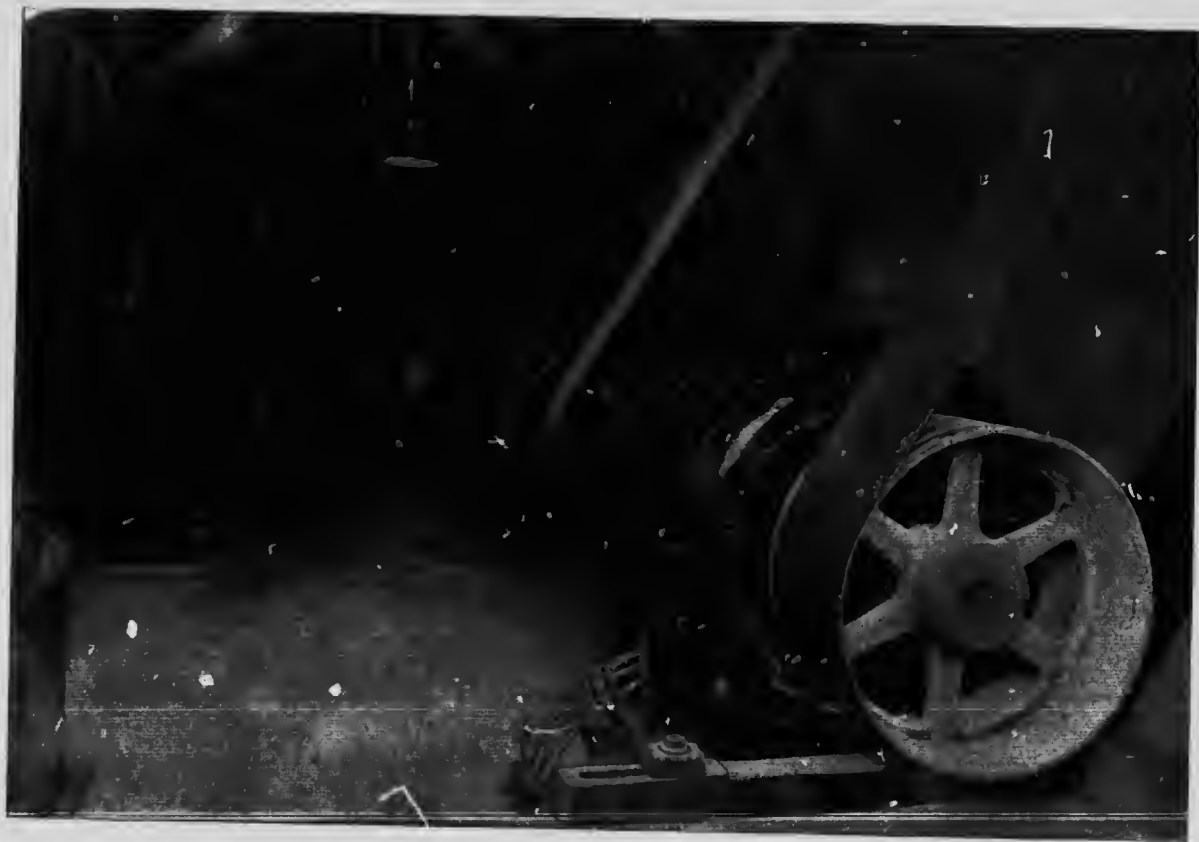
AMALGAMATED ASBESTOS CORPORATION LIMITED - MOTOR ROOM, BRITISH CANADIAN MILLS
