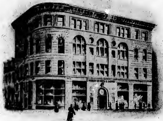
HENRY BIRKS & SONS' BUILDING, MONTREAL
