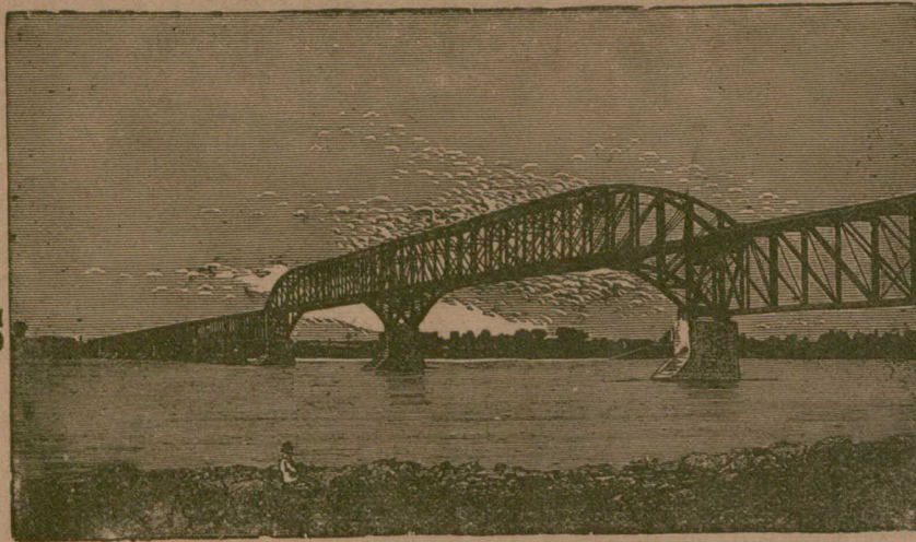
ST. LAWRENCE RIVER BRIDGE CANADIAN PACIFIC RAILWAY, LACHINE, P. Q.
