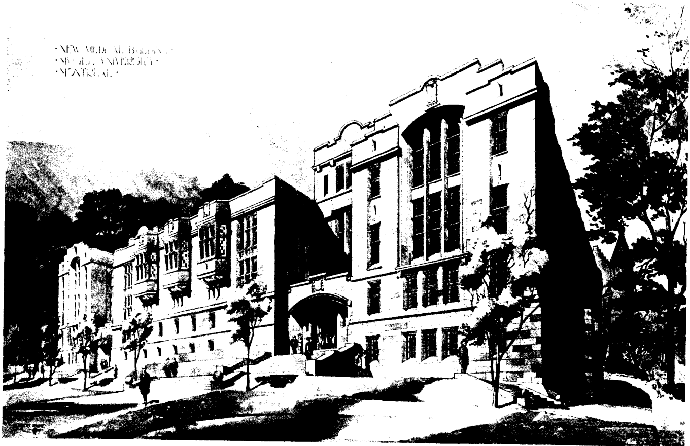
McGill College Buildings, Equipped with Otis Elevators
