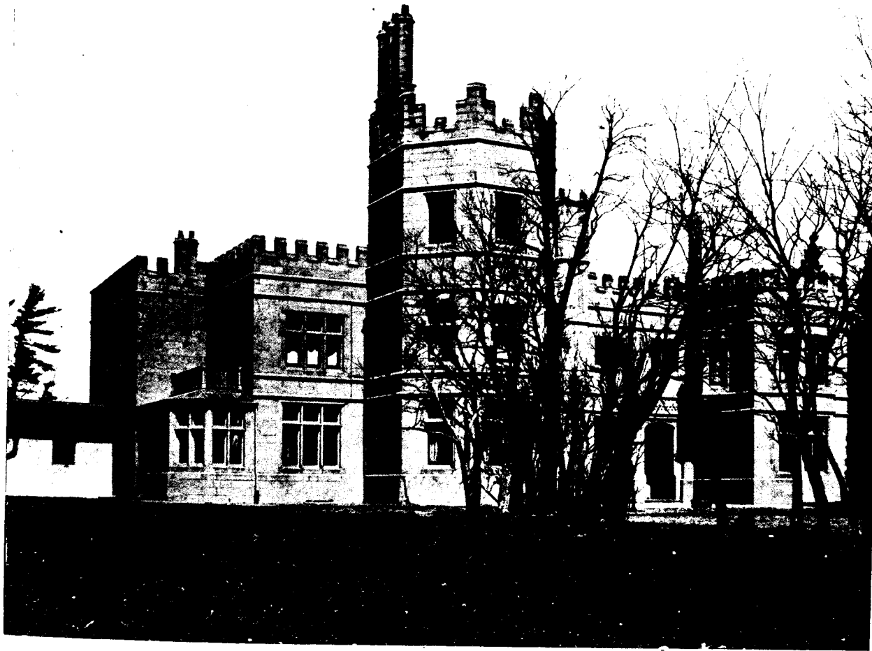
Residence of Mr. A. Ansley, at Glen Grove, Eglinton. Geo. W. Gouinlock, Architect.
