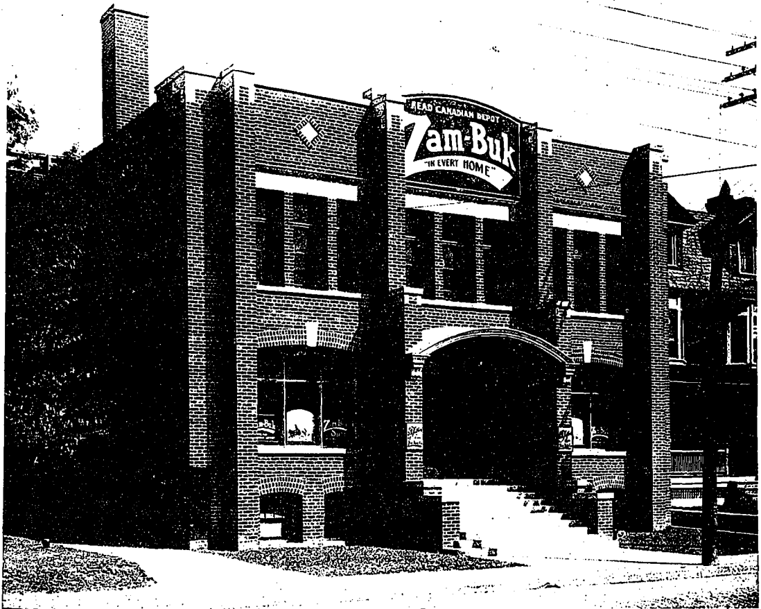
Zam-Buk Warehouse, Toronto, Ontario. Wickson & Gregg, Architects.
