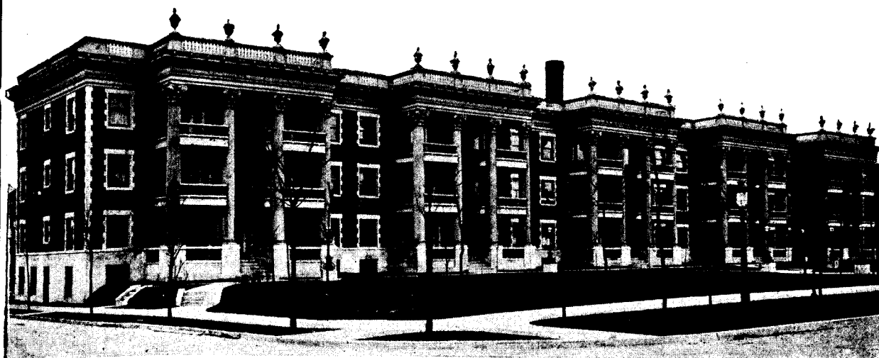
"Colnade" Apartments, Kansas City, Mo. Sellers & Marquis, Roofers. J. W. McKecknie, Architect
