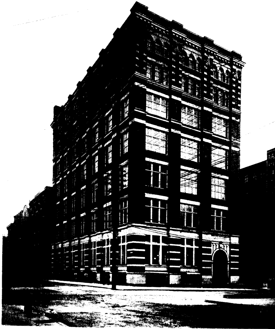
Ogilvie Building, Toronto. Burke, Horwood & White, Architects. Witchall & Son, Contractors.
