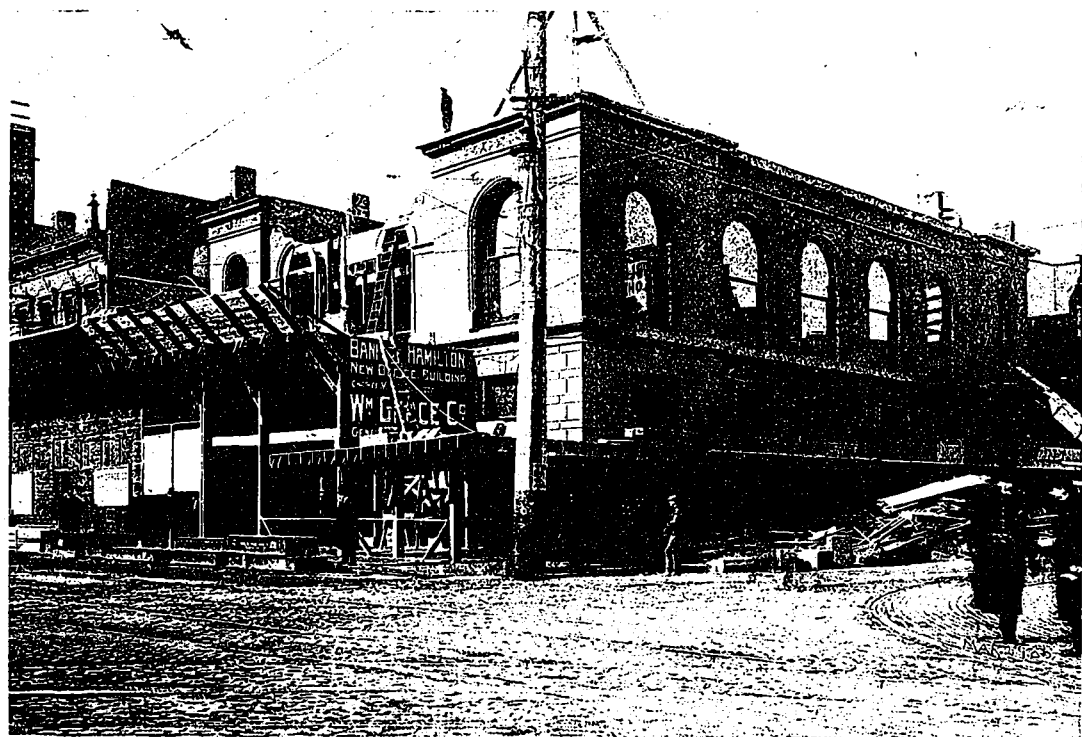
Preserved Portion of Walls of Old Building. Bank of Hamilton, Head Office, Hamilton, Ontario. Charles Mills, Architect.
