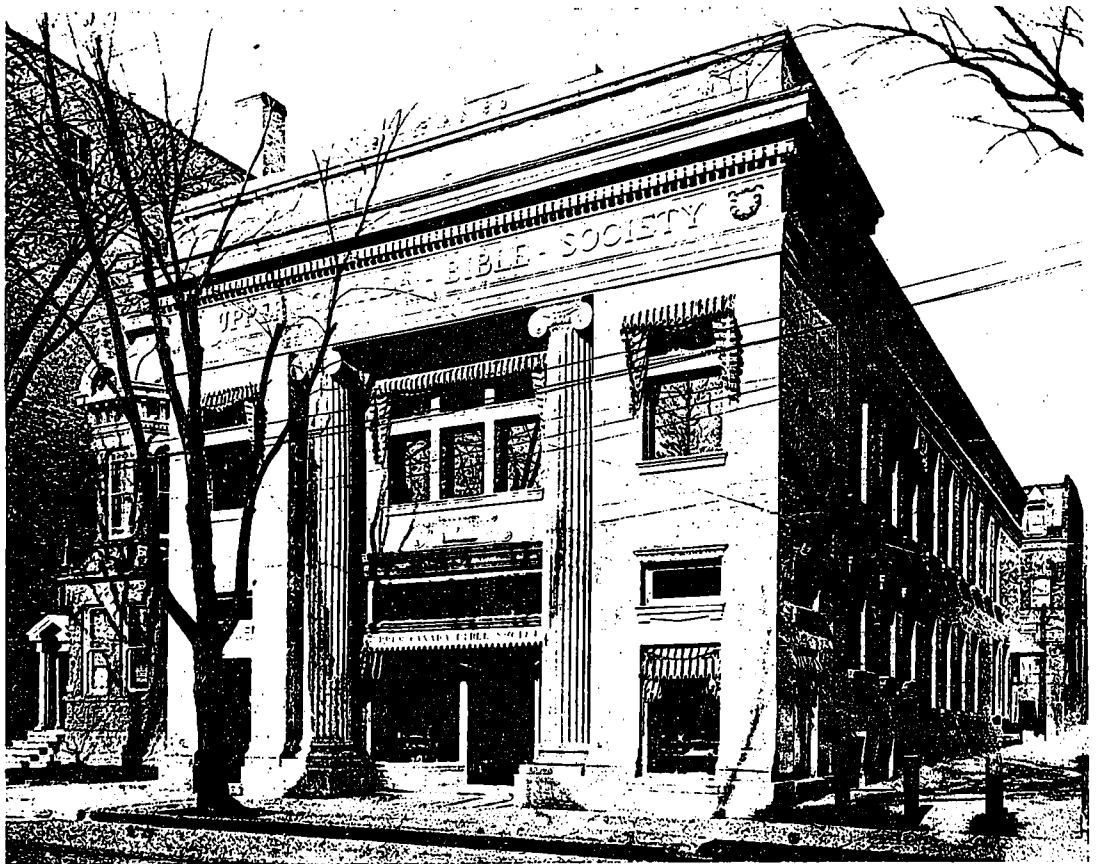
Upper Canada Bible Society Building, Toronto, Ontario. Gordon & Helliwell, Architects.
