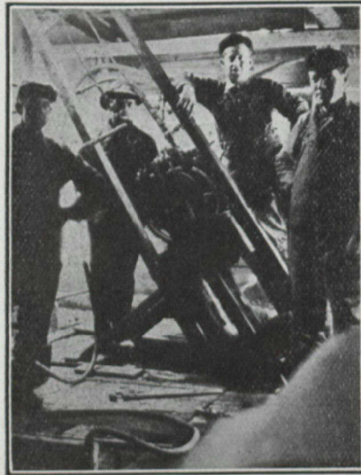
A Terry Class A Drill working at an angle of 45° on the West Dome Mine, Porcupine.
