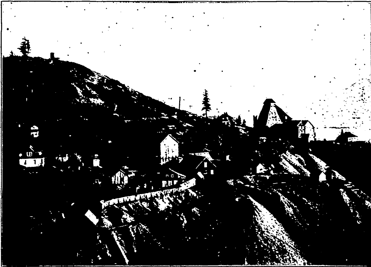
Le Roi No. 2 Co.'s Josie Mine Surface Works and Dumps.—Le Roi Head Works over Combination Shaft in Background.
