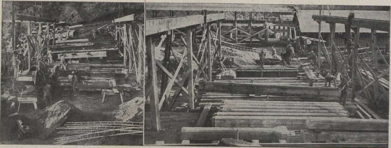
Views of Casting Floor Showing Concrete Mixer and Telpher Track.
