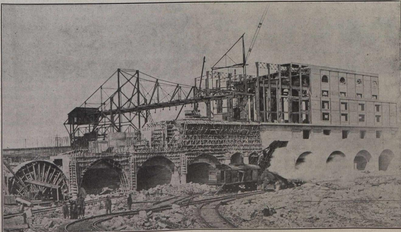
Down-stream Face of Cedars Rapids Power House, Showing Method of Construction, and the 84-foot Boom.
