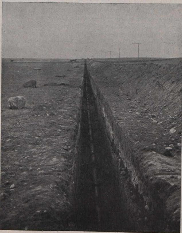
Fig. 2.—Excavated Ditch, Showing Some of the Boulders Moved by Machine.
