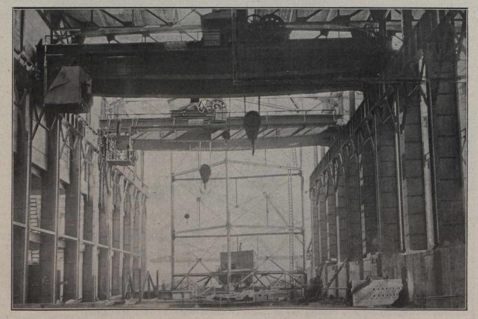
Interior View of Power House During its Construction, Showing Crane Service for the Installation of Machinery.
