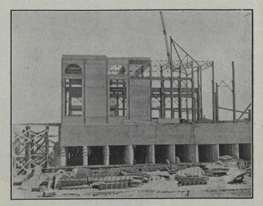
Showing Construction of the Walls of the Transformer House. (Unit Construction Method.)
